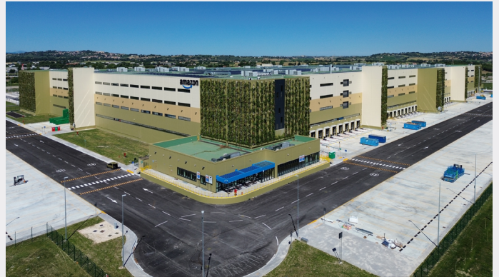
JESI (AN) LOGISTICS HUB A0L1: Development of a logistics hub comprising a multi-storey warehouse of 232,500 sq m distributed over four levels, designed for robotised storage. The facility is equipped with 70 loading bays. The building is BREEAM EXCELLENT certified.
