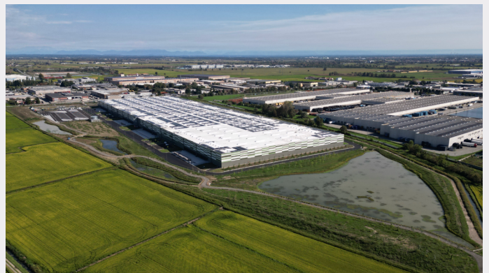
SAN PIETRO MOSEZZO (NO) LOGISTICS HUB: Development of a logistics hub consisting of two buildings: Building A (60,000 sq m, including approximately 1,500 sq m of office space and 51 loading bays) and Building B (100,000 sq m, including approximately 7,500 sq m of office space and 85 loading bays). The development is LEED Platinum certified.
